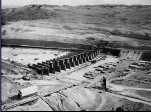
Fort Peck Dam - Biggest Public Works Administration project
